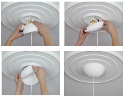
Installation of the rubber CableCup.
